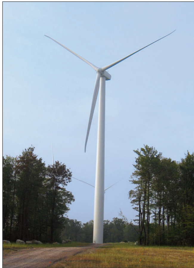
Figure 2. A wind turbine shown in a “feathered” position during the curtailment experiment at the Casselman Wind Project in Somerset County, south-central Pennsylvania.
