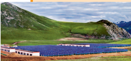
2 MW Hydro/PV Generating System in Yushu, Qinghai Province, China
