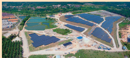
8 MW PV on landfill, Pajam, Malaysia
