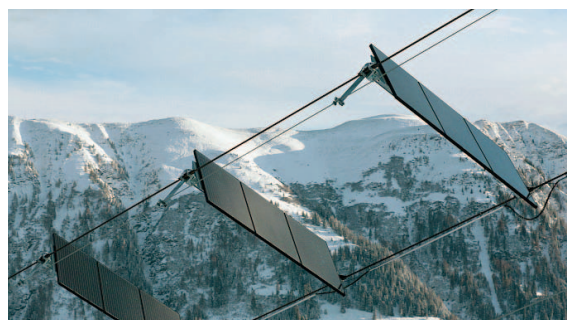
Solar powered ski-lift in Tenna, Switzerland, courtesy Solarskilift.ch
