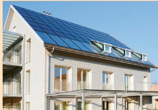
PV and solar thermal combined on a Swiss house, courtesy SOLTOP AG
