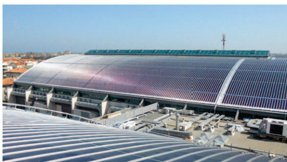
Green Utility SpA-owned Si-a 4,3 MWp PV plant, Rimini Fair, by the contractor Acea Arse SpA
