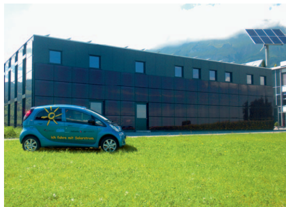
Solarpark Gams, facade integrated PV, Courtesy Heizplan AG, Switzerland
