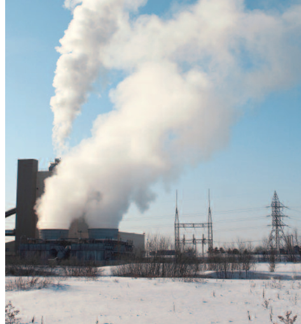
PHOTO Despite the fact that this 20MW power plant claims to be a Combined Heat-and-Power facility, the St-Felicien cogeneration plant does not distribute its heat to surrounding installations and wastes about 75% of the potential energy to heat and pollutants.
