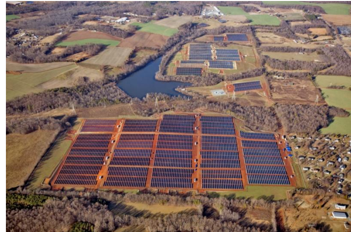
Duke Energy 15.5 MW Davidson PV Project (Courtesy: SunEdison)
