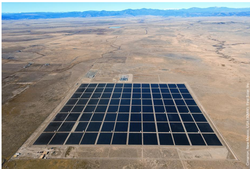
Tri-State G&T Cimarron 30 MW PV Project (Courtesy: First Solar)
