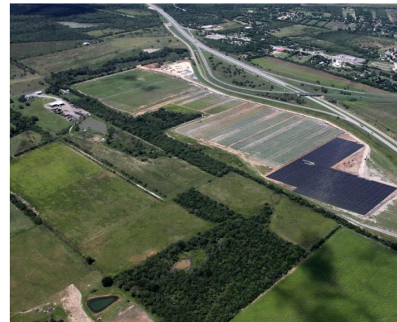
CSP Energy 14.5 MW Blue Wing PV Project (Courtesy: Juwi Solar)
