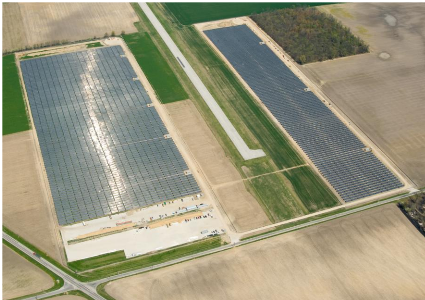
Ohio Power 10.1 MW Wyandot Solar Farm (Courtesy: PSEG Solar Source LLC)
