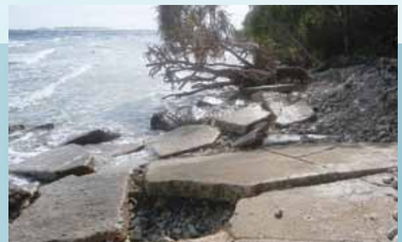
Erosion on atoll islets has undermined and damaged infrastructure built during WWII. (Source: C. Fletcher)
