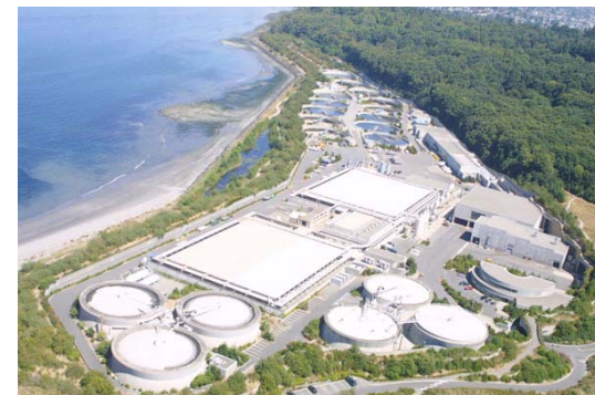
West Point Treatment Plant Seattle, Washington
