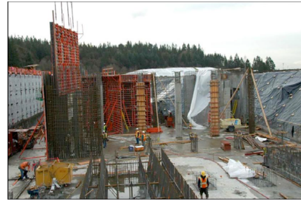
Brightwater Treatment Plant construction
