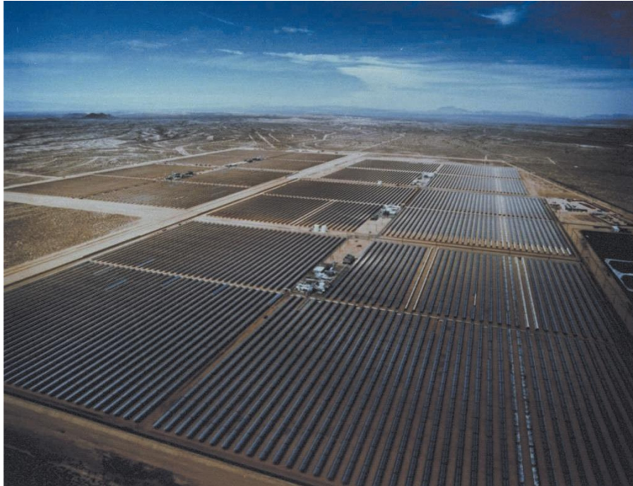
Figure E.1: SEGS III–SEGS VII Solar Plants at Kramer Junction, California
