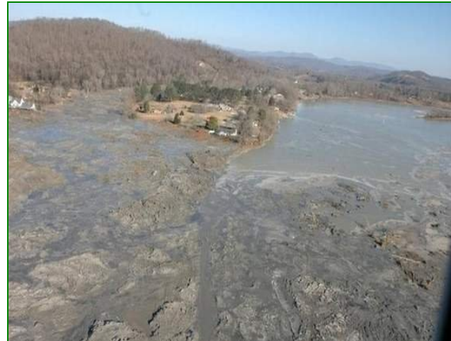
Aerial photo of the Dec. 22 coal ash spill in Tennessee
