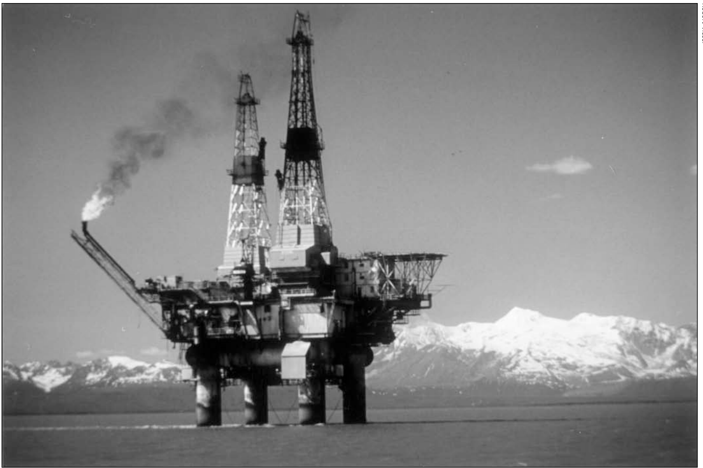
Chevron's Steelhead Platform, Cook Inlet, Alaska
