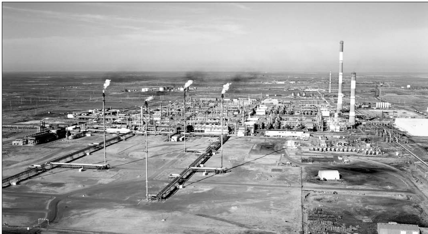
Flaring and sulfur pads at the Chevron/Tengizchevroil Tengiz Field in western Kazakhstan.
