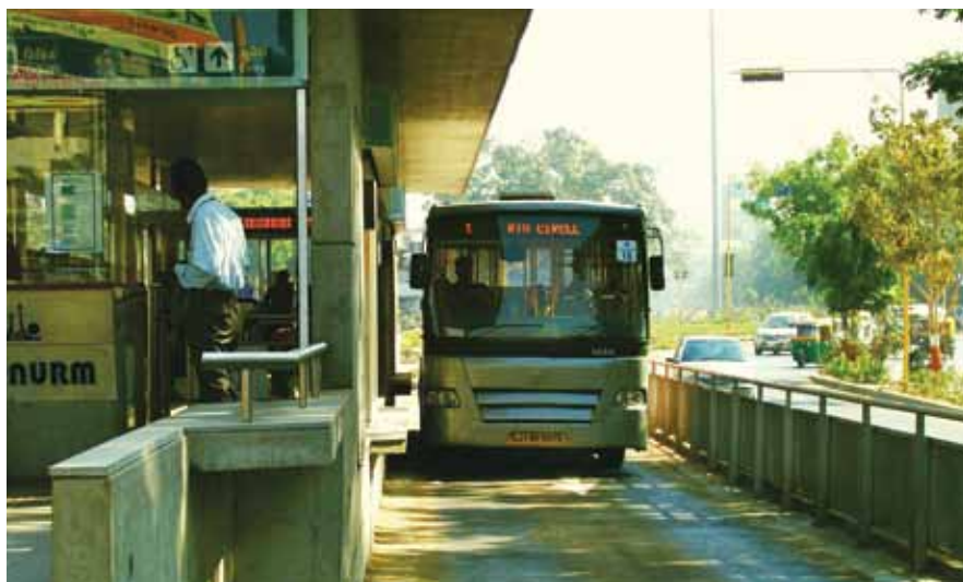
Left: Janmarg stations have pre-paid boarding. Image: Chris Kost. Opposite: At night, Janmarg stations are well-lit for passenger safety. Image: Shreya Gadepalli
