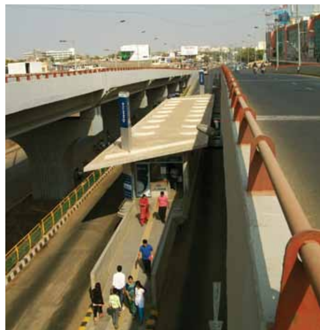
Above: Passengers board Janmarg at-grade, a vast improvement on the narrow, treacherous steps of AMTS buses. Below: The city built split overpasses to allow the BRT system to remain on the street level. Images: Shreya Gadepalli
