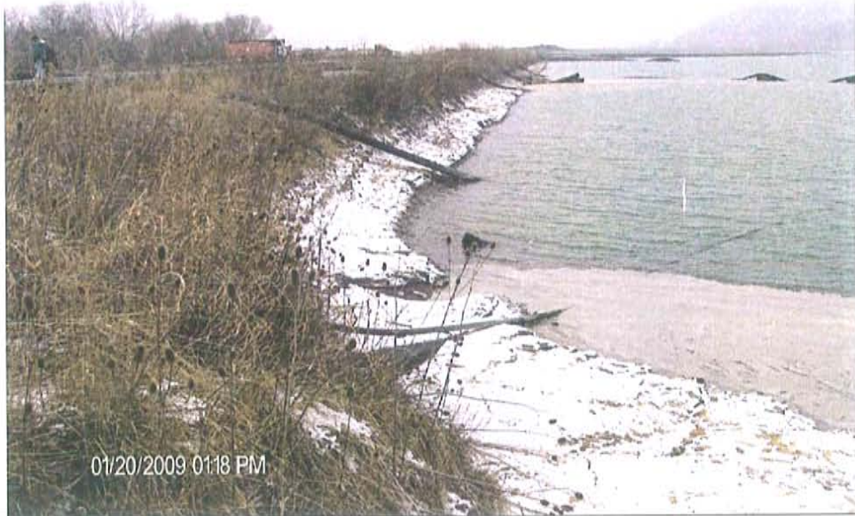
Photo #9: West embankment, upstream slope, looking North
