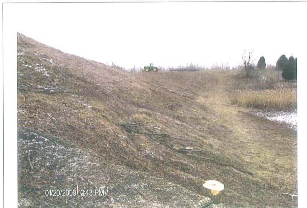
Photo #14: North embankment, shared dike with emergency ash pond, looking West
