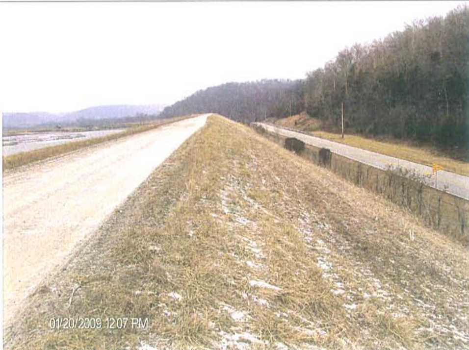
Photo #4: East embankment, crest and downstream slope, looking North
