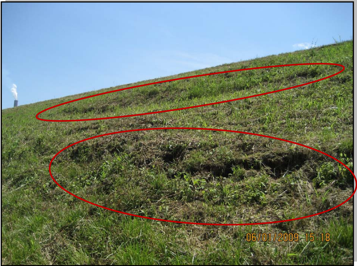
Photo 13 – Old slough on eastern downstream slope
