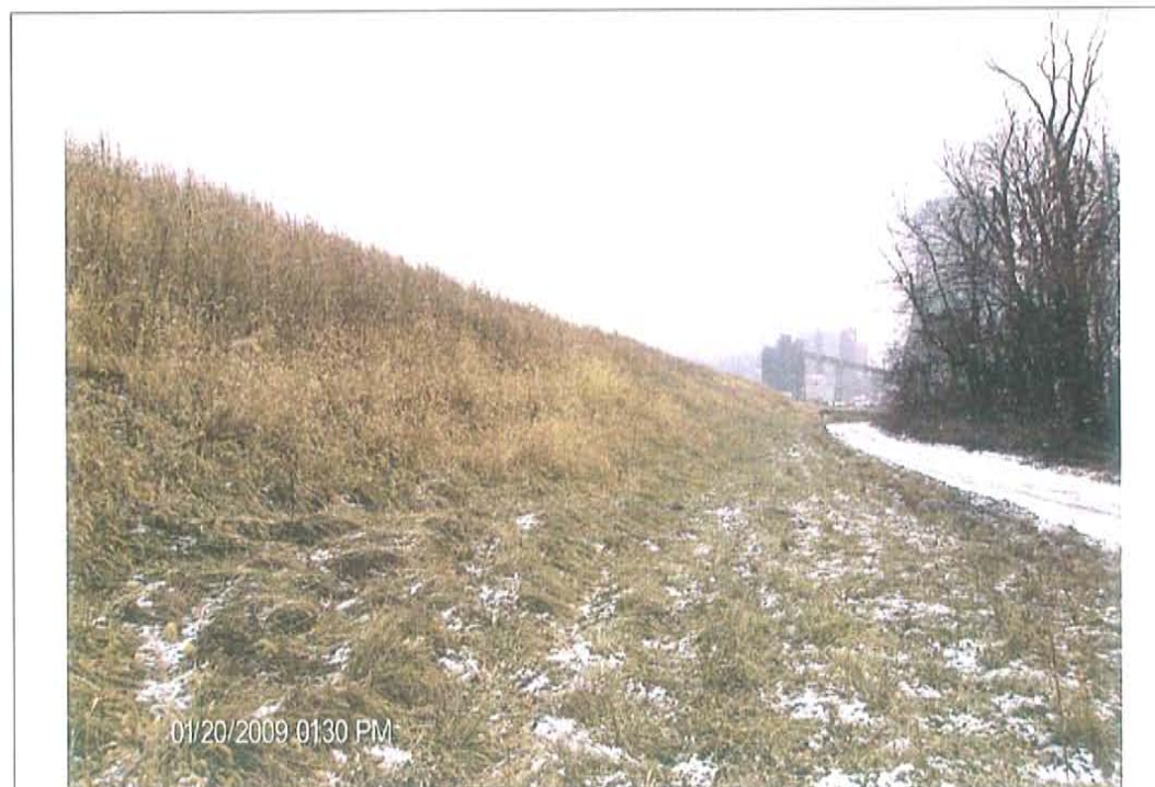
Photo #12: West embankment, downstream slope and toe, looking South
