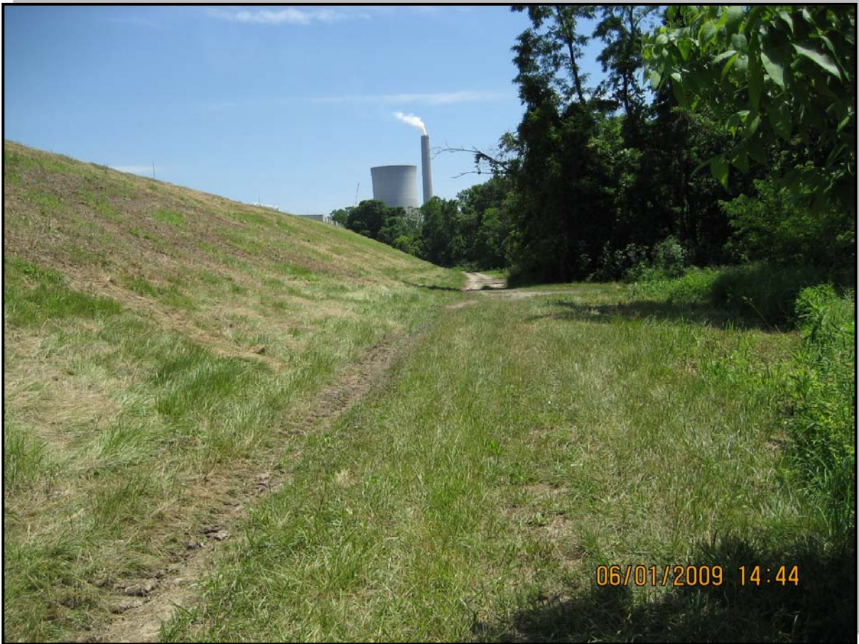
Photo 11 – View along toe of western downstream slope looking south
