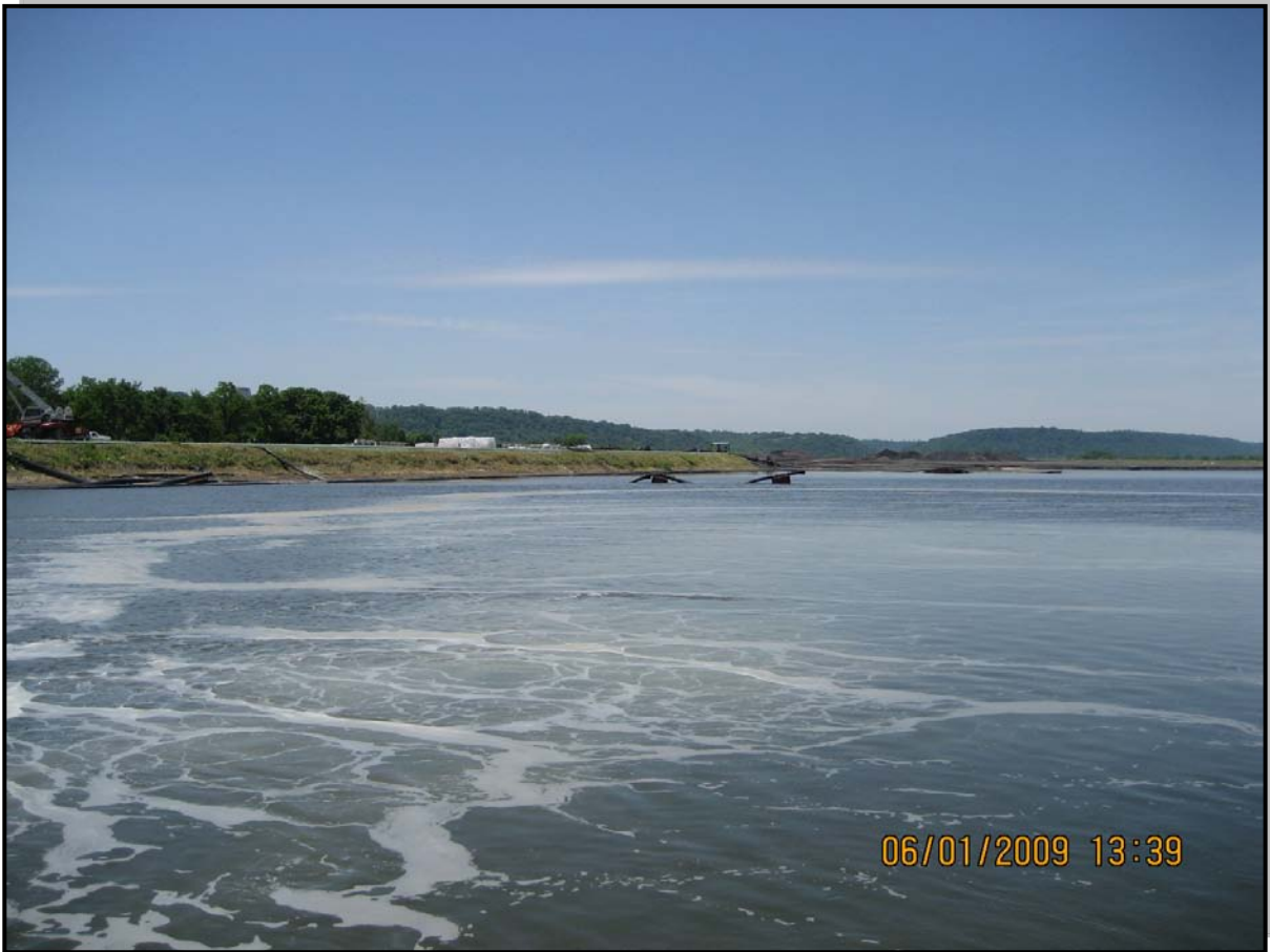
Photo 3 - Typical overview of impoundment viewed from Floating Dock along South Dike
