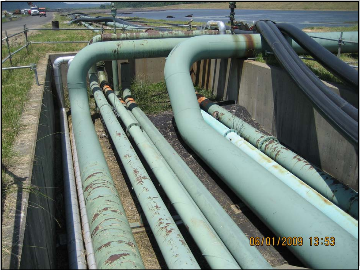
Photo 5 – View of influent/effluent piping and vault along west embankment crest
