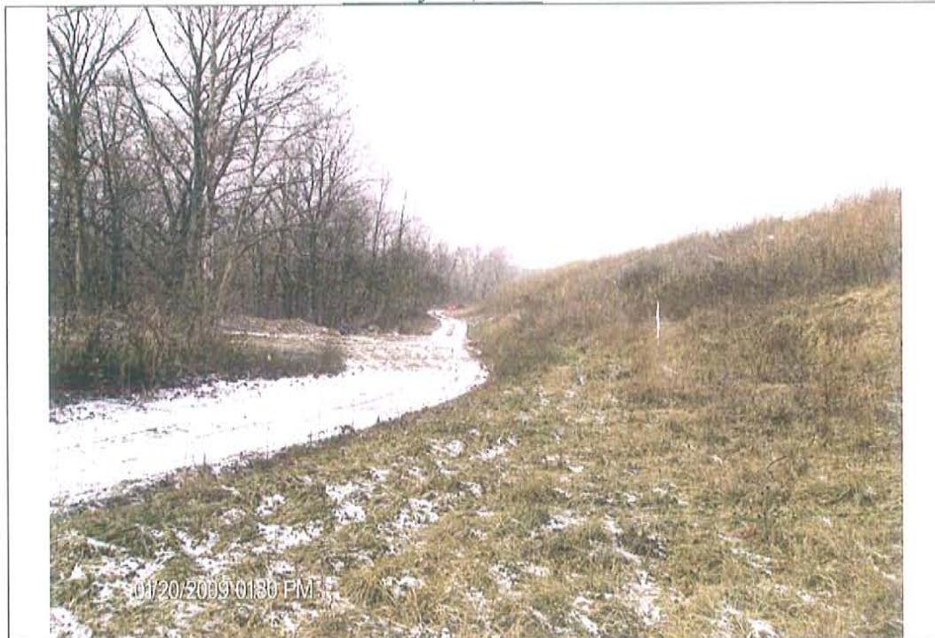
Photo #11: West embankment, downstream slope and toe, looking North
