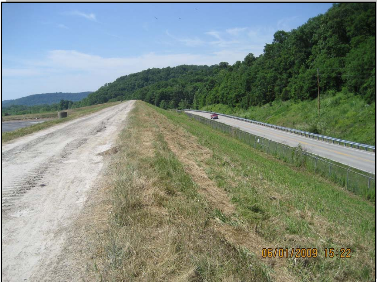
Photo 14 – View along crest and upstream slope of eastern embankment looking north
