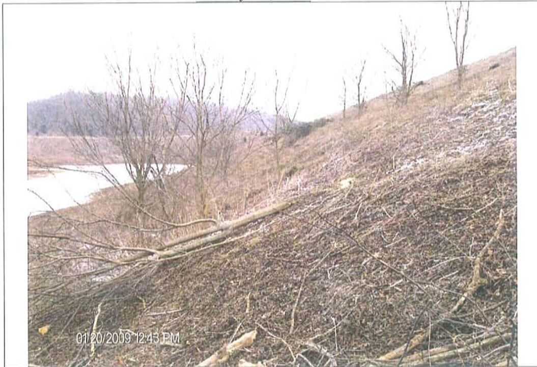
Photo #13: North embankment, shared dike with emergency ash pond, looking East
