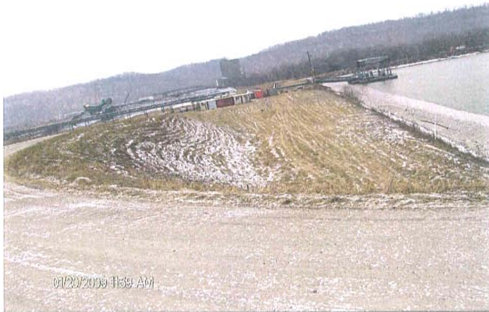
Photo #3: South embankment, upstream slope, looking West
