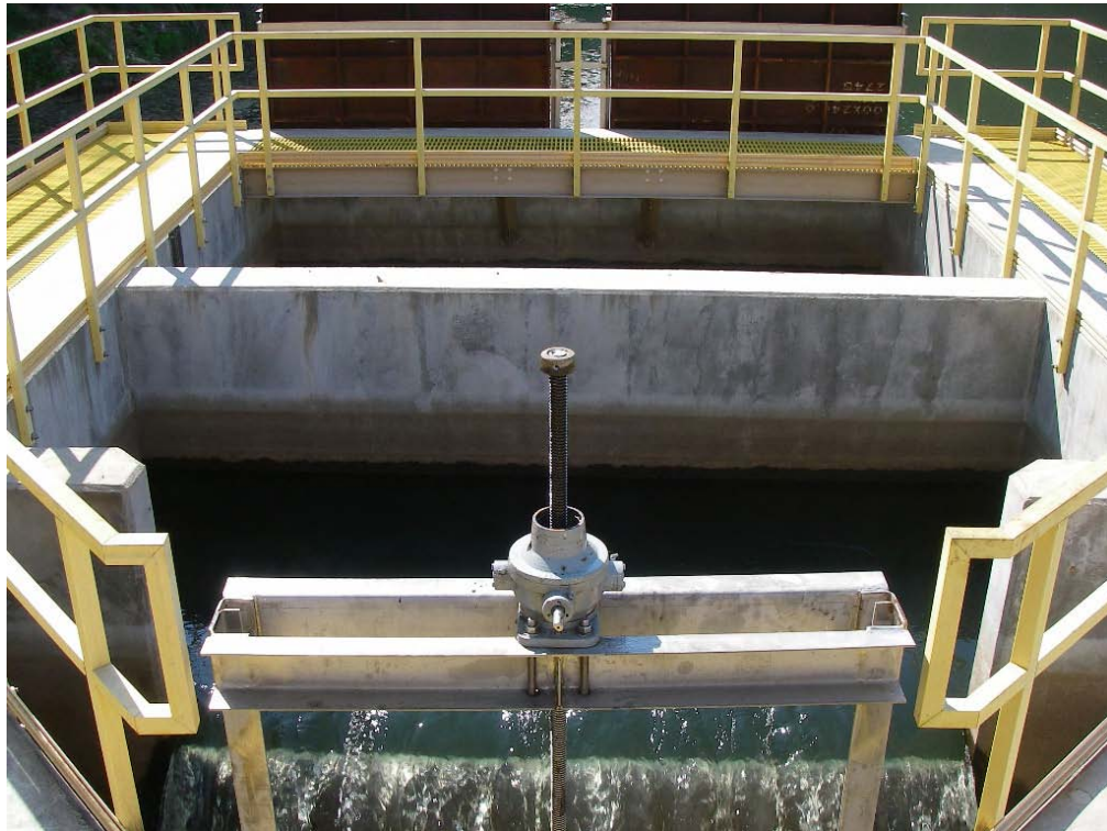
PHOTO 2: CLOSEUP OF WEIR INTAKE
