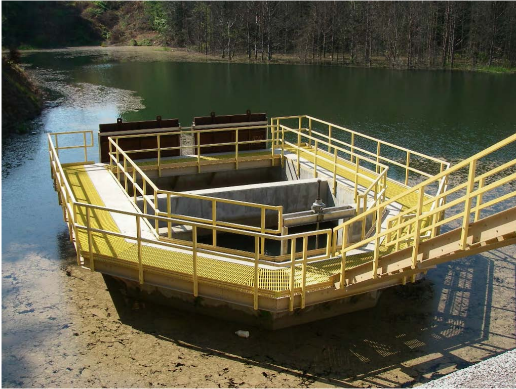
PHOTO 1: RATTLESNAKE DAM WEIR FLOW INTAKE STRUCTURE
