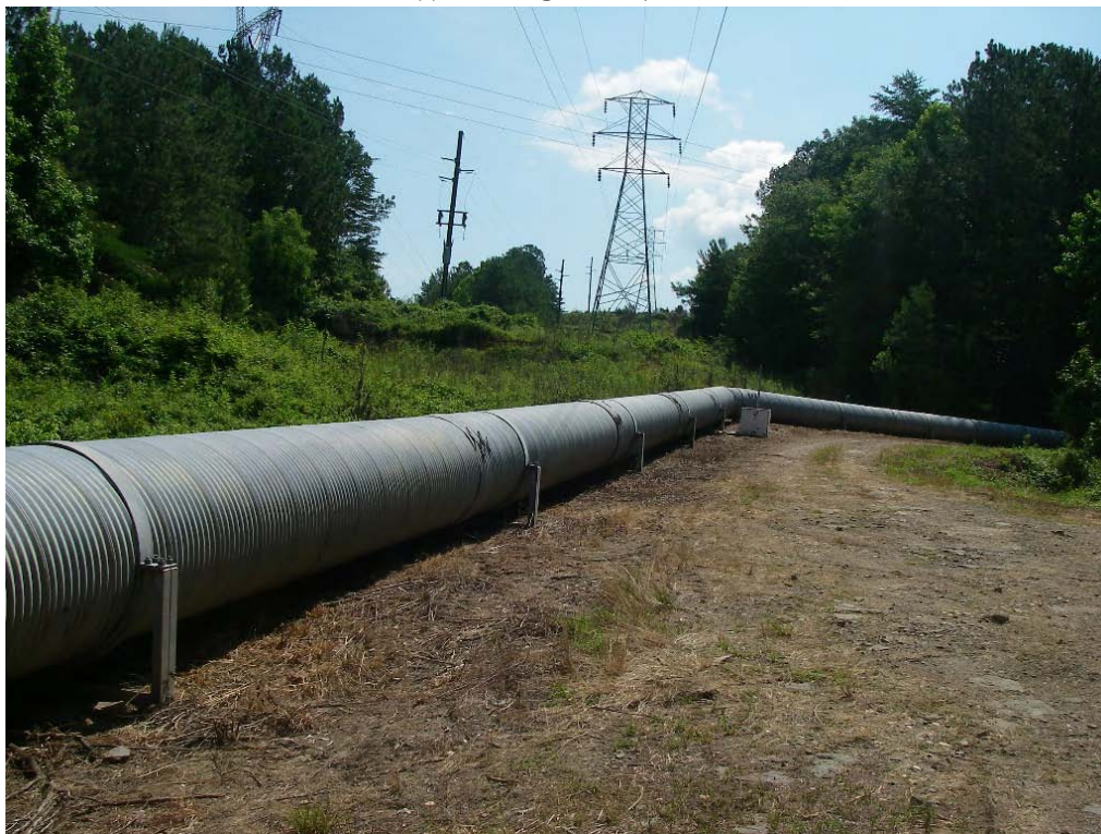
PHOTO 27: DISCHARGE LINE FROM RATTLESNAKE DAM TO BLACK WARRIOR RIVER
