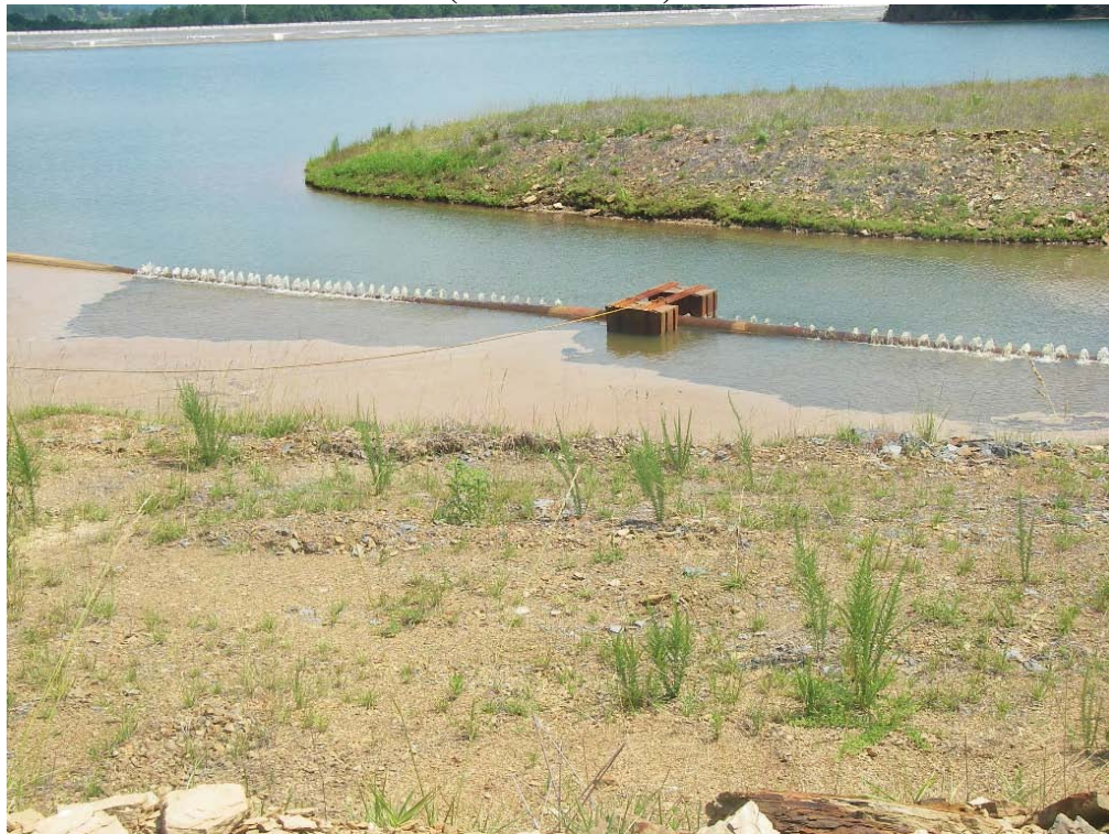
PHOTO 32: BUBBLER AERATION LINE AT INTERMEDIATE DIKE (LOOKING E)
