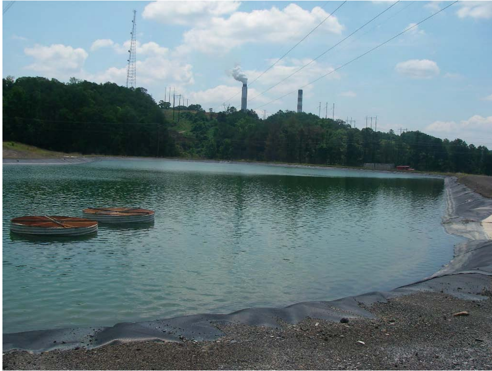
PHOTO 35: DECANT PIPES IN SEDIMENT BASIN
