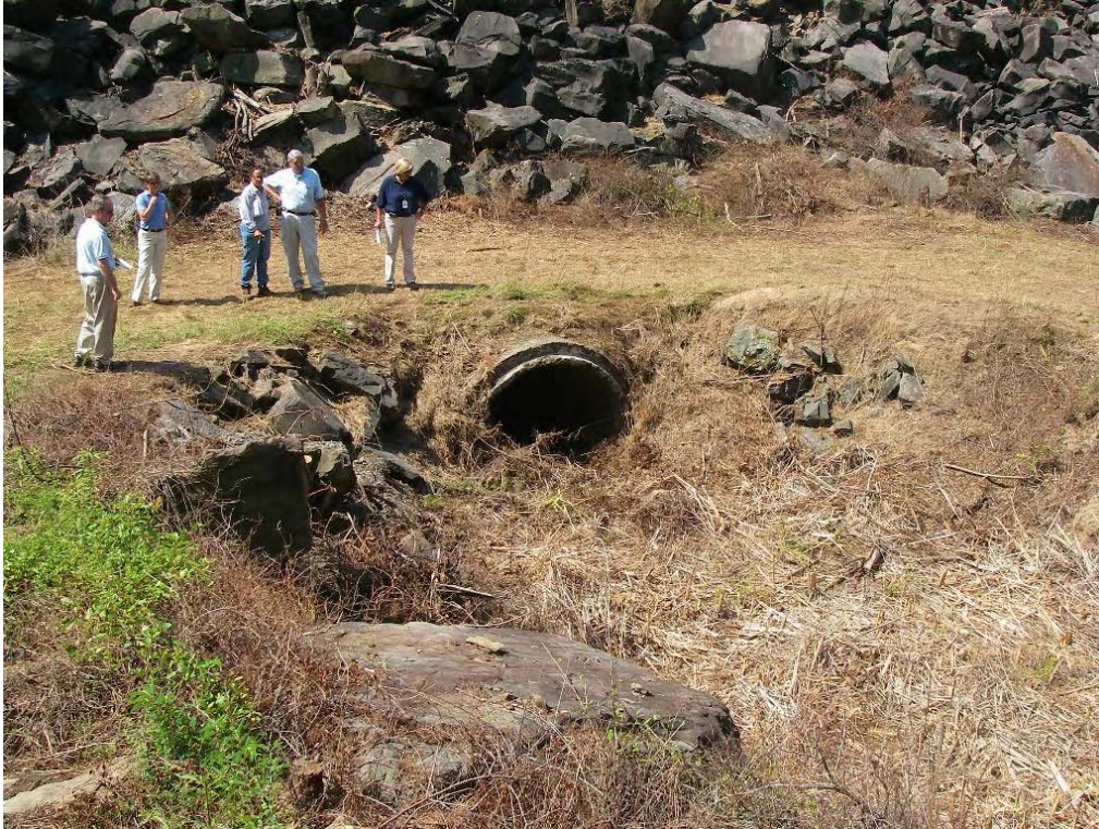
PHOTO 15: ORIGINAL BYPASS CHANNEL & CULVERT (ABANDONED, LOOKING S)
