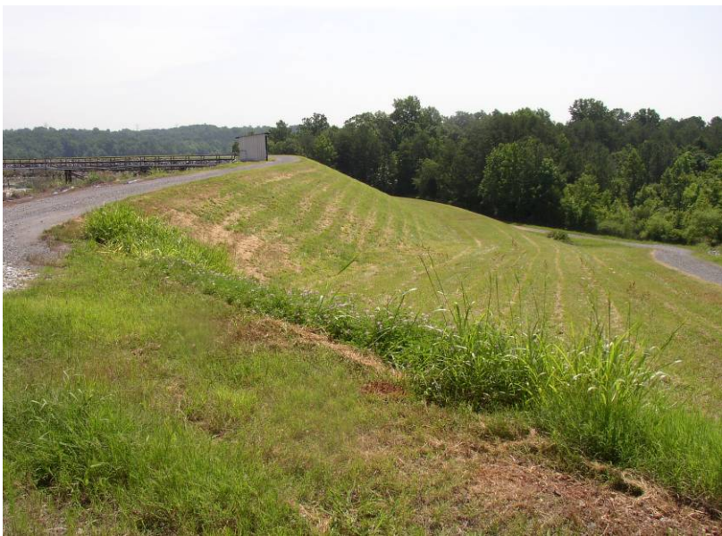
# 1 Southern Crest & Downstream Slope of East Dike – Local Reseeded Area
