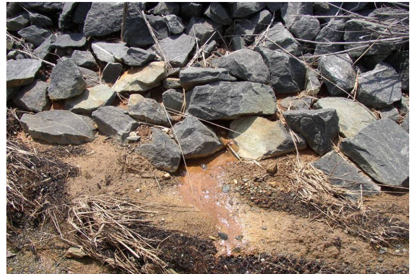
#34 Minor Local Clear Seepage Discharges from Downstream Rock Toe at South End of East Dike
