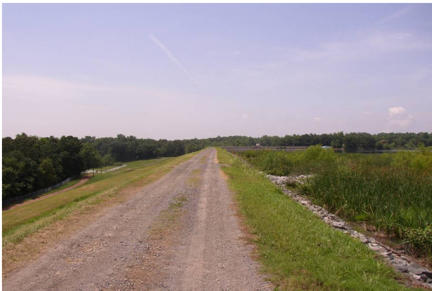
#15 Crest of East Dike Looking South - Satisfactory Alignment
