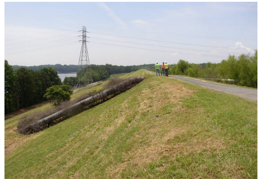
#17 Northern Portion of Downstream Slope of East Dike
