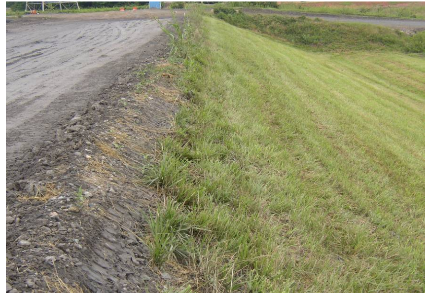
#62 Crest of Western Portion of North Dike
