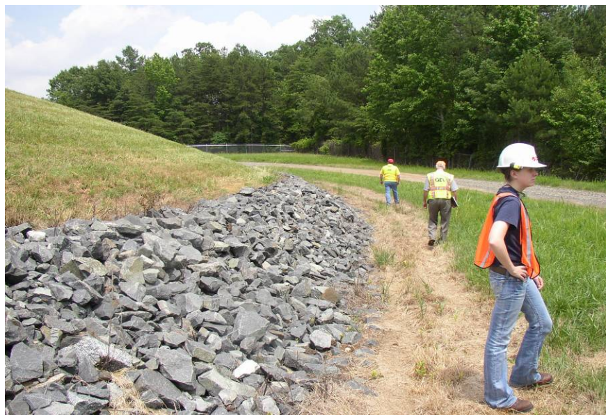
#28 Riprap at Downstream Toe of East Dike - Southern Portion
