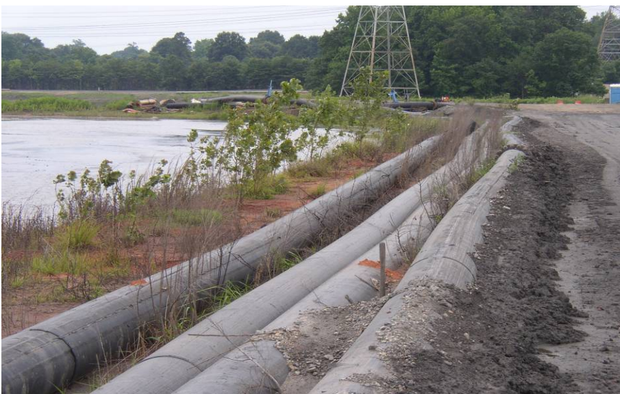
#50 Pipes Used for Sluicing
