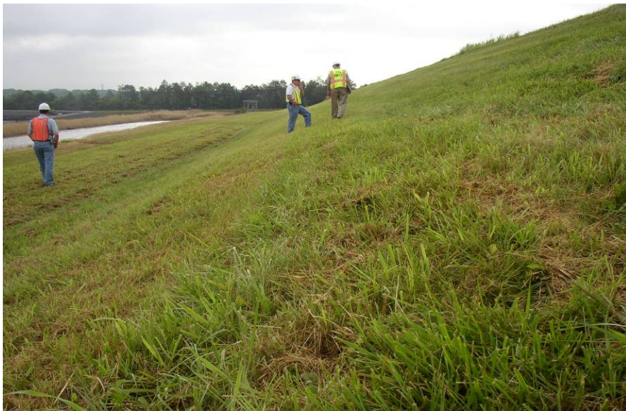
#53 Downstream Slope of North Dike (Central Area)
