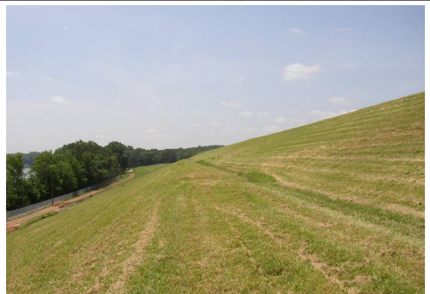
#22 Stability Berm and Downstream Slope of East Dike
