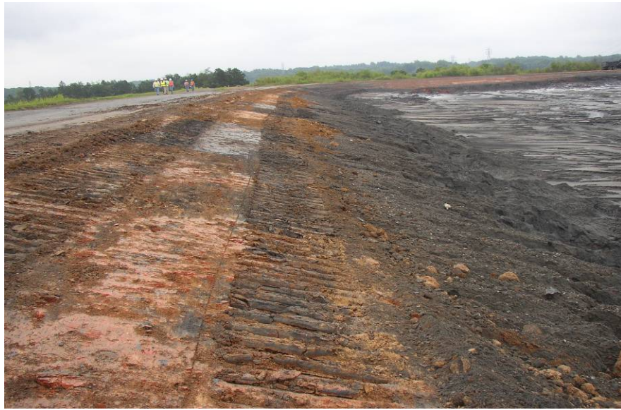
#60 Dewatered Cell 3, Ash Excavated to up to 20-Foot Depth
