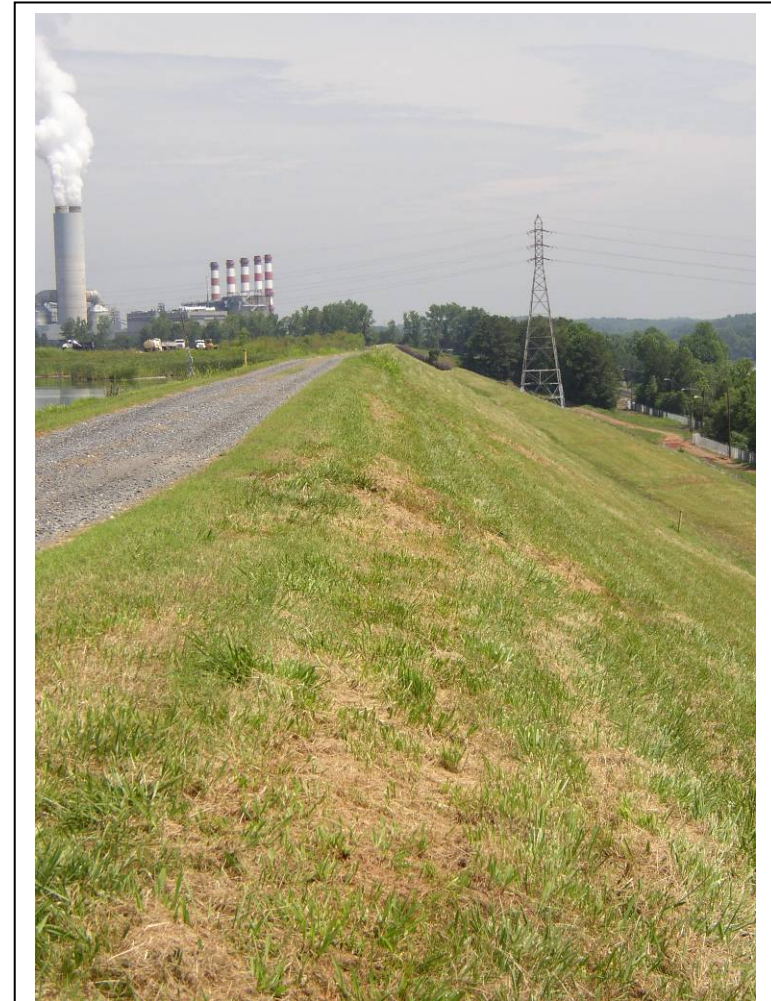
#6 Crest & Downstream Slope of East Dike
