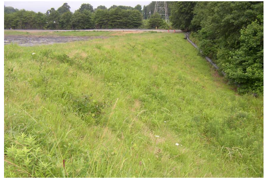
#70 Downstream Slope Near Western Limit of North Dike
