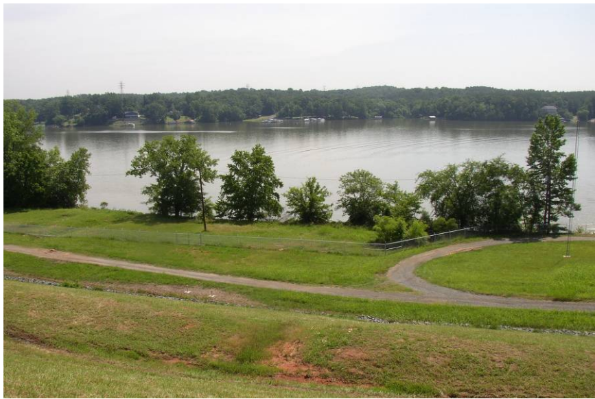
#7 Downstream Berm & Toe Area of East Dike – Southern Portion Lake Wylie at Downstream Toe
