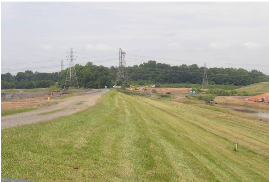
#20 Overview of Central Portion of North Dike
