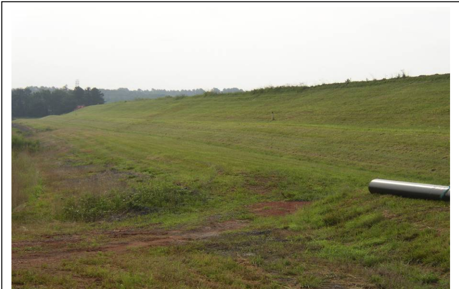
#52 Overview of Downstream Slope from a Point Near Construction Ramp
