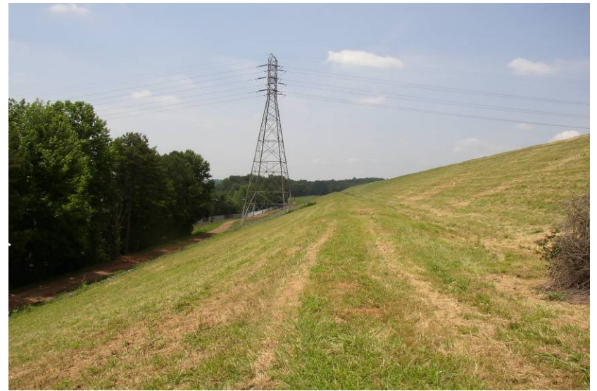
#21 Stability Berm at North End of East Dike
