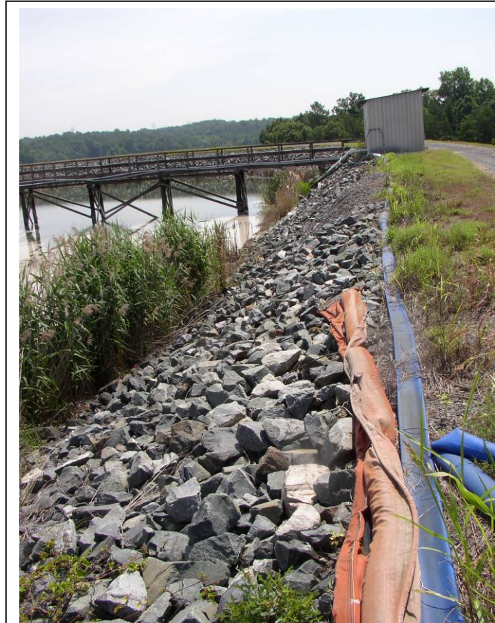
#3 Upstream Slope & Bridge to Drop Inlet Structure
