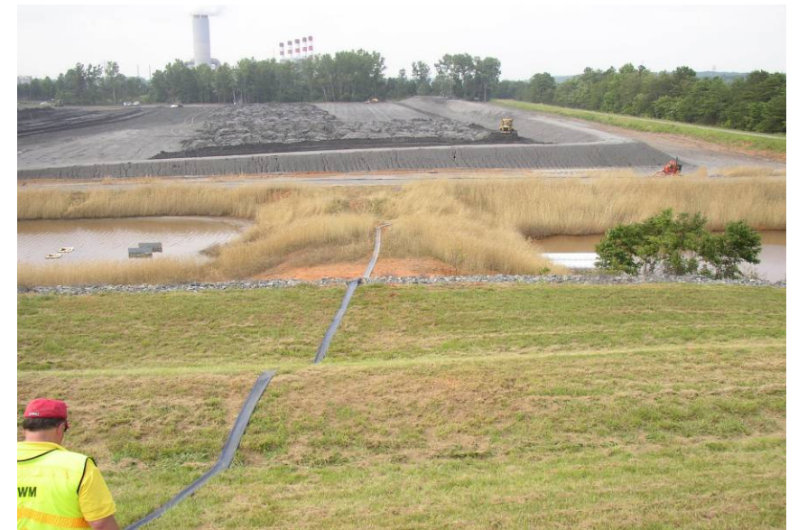
#43 Stabilizing Berm from Crest
