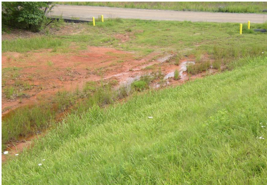
#69 Ponded Surface Drainage & Seepage Near Transmission Tower at West End of North Dike
