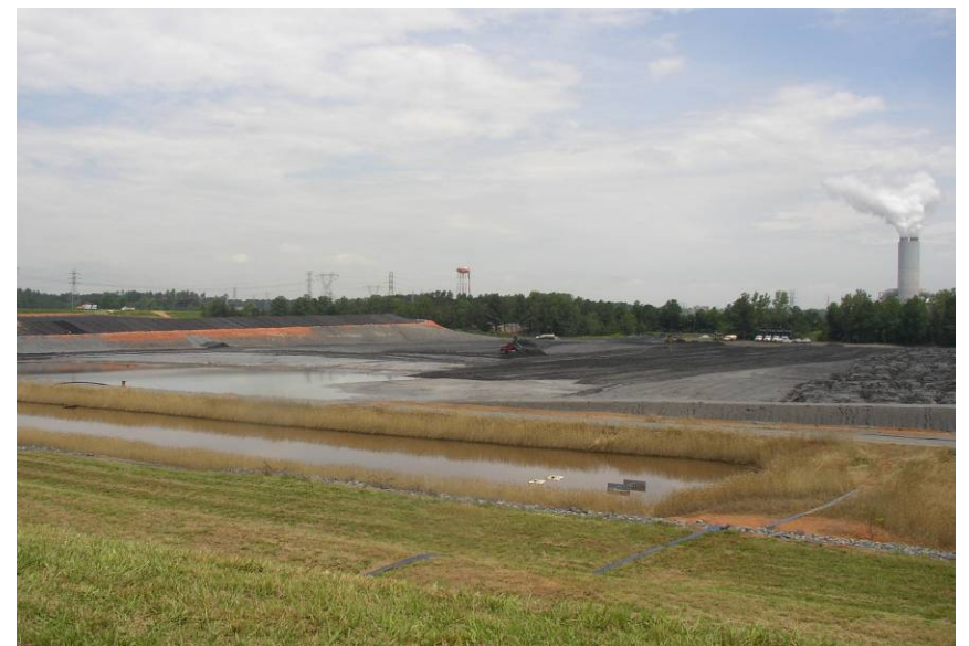
#18 New Ash Landfill Construction
