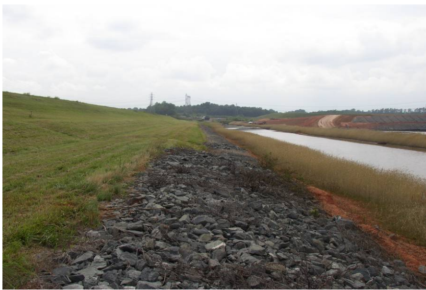
#45 Downstream Toe of North Dike
