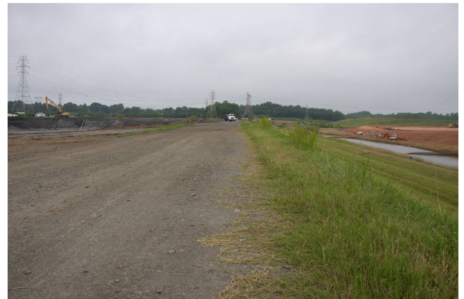
#56 Widened Upstream Crest (to 45 Feet) to Create Haul Road
