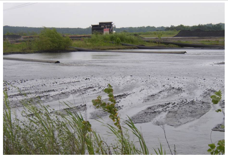
#48 Inlets of Sluice Pipes - Pool Elev. 635 +/- in Cell 2
