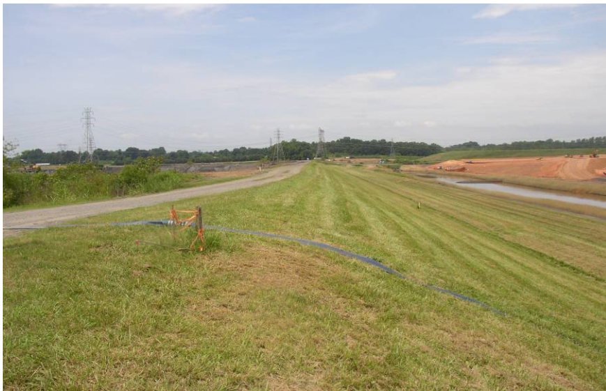
#19 Overview of Crest & Downstream Slope of North Dike
