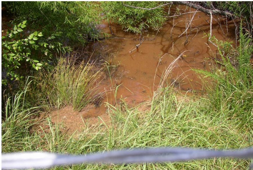
#32 Poned Surface Water East of Downstream Toe Near Outlet
