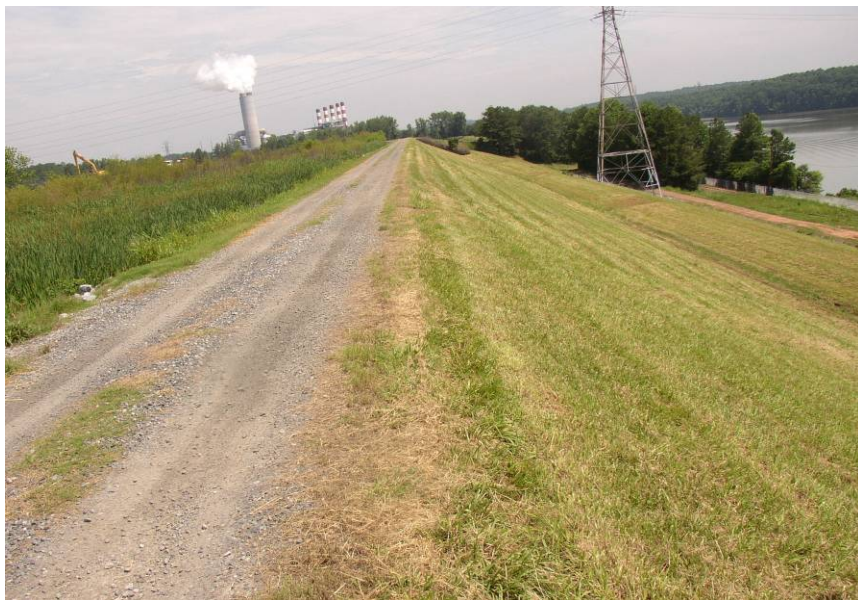
#12 North End of East Dike: Cell No. 3 Note Cell is Full to Design Grade – Elev. 640 or above
