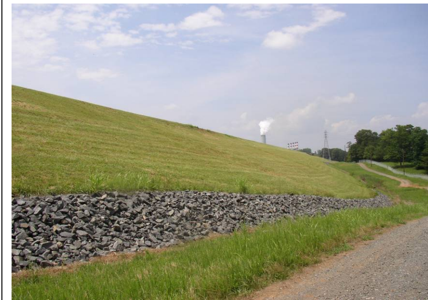
#30 Overview of Downstream Toe of East Dike Near Maximum Section
