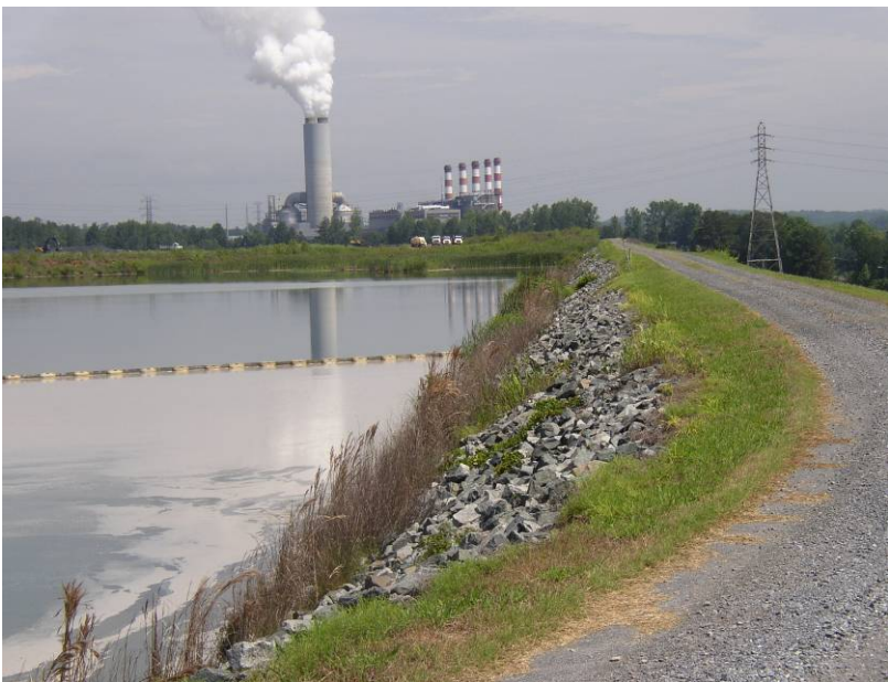
#5 Overview of Crest & Upstream Slope of East Dike – Polishing Cell
