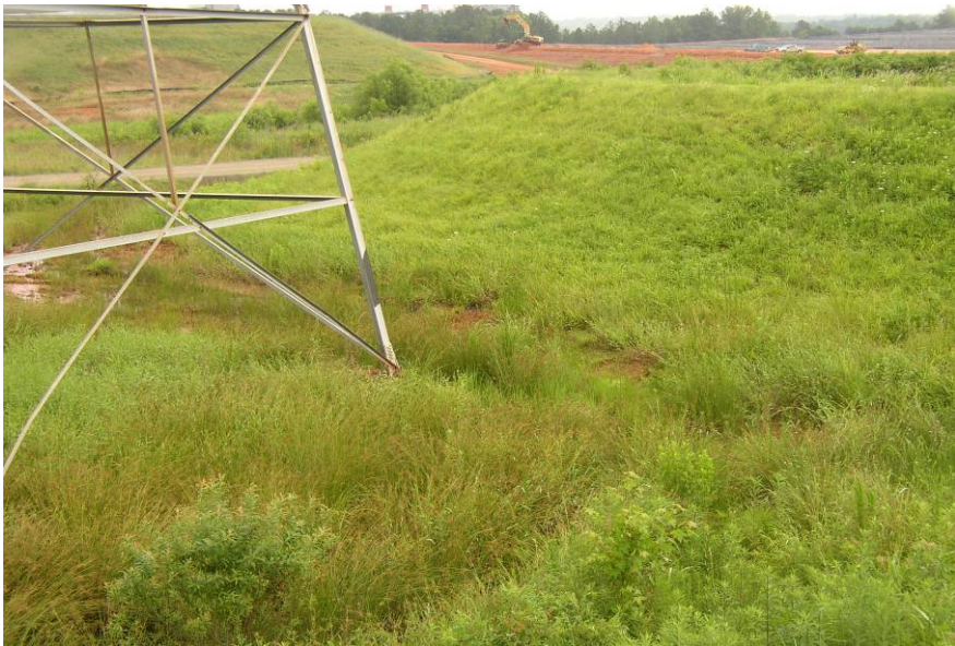
#72 Area to Improve Drainage at West End of North Dike
