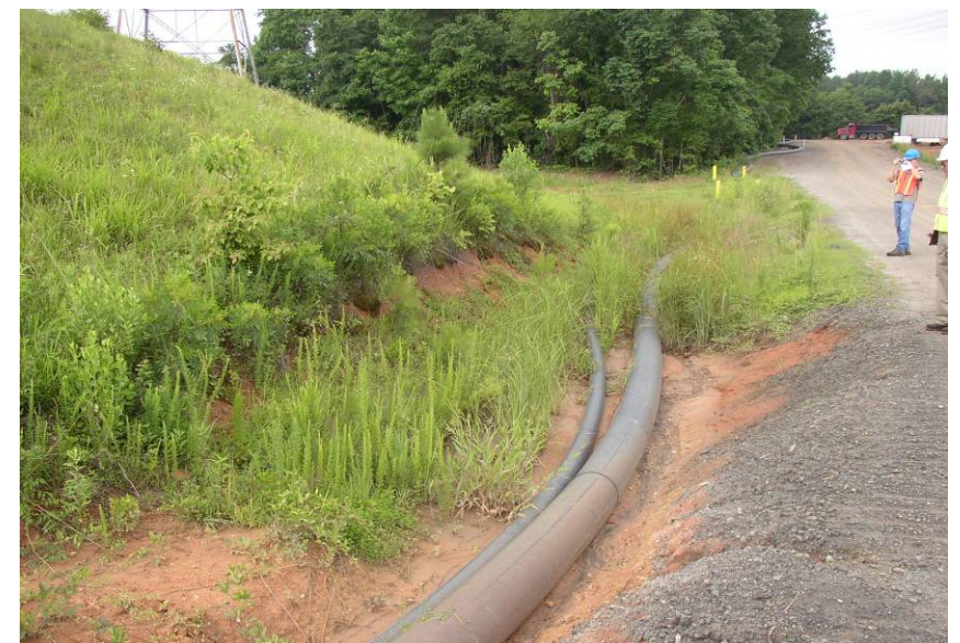
#75 Cut Into Downstream Toe of North Dike For Pipe Installation
