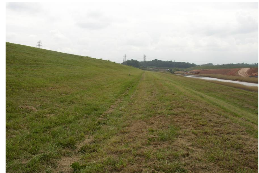
#44 Upper Berm of North Dike - 15 Feet Wide @ Elev. 630
