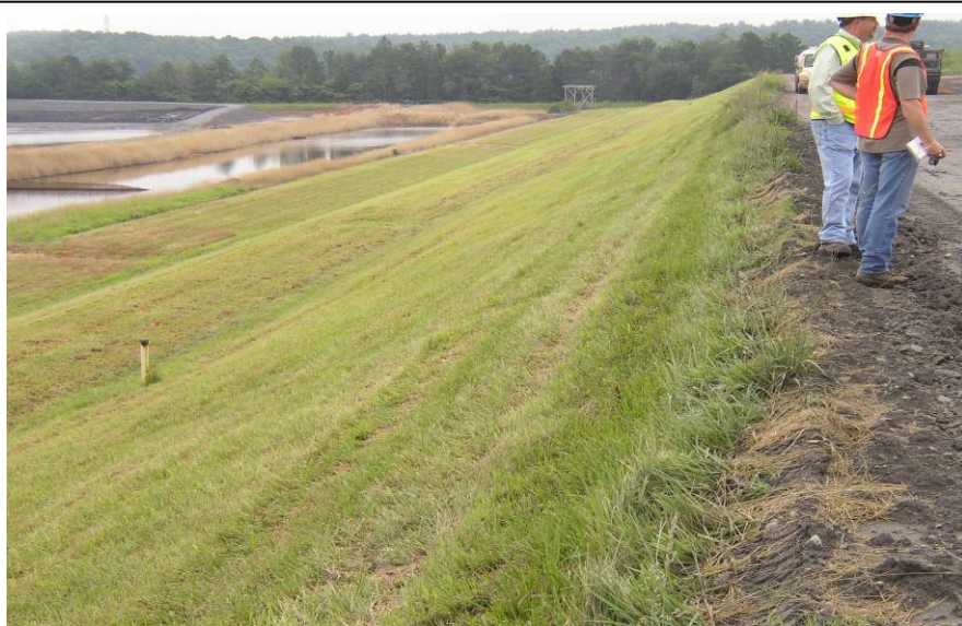
#61 Overview of Central Portion of North Dike
