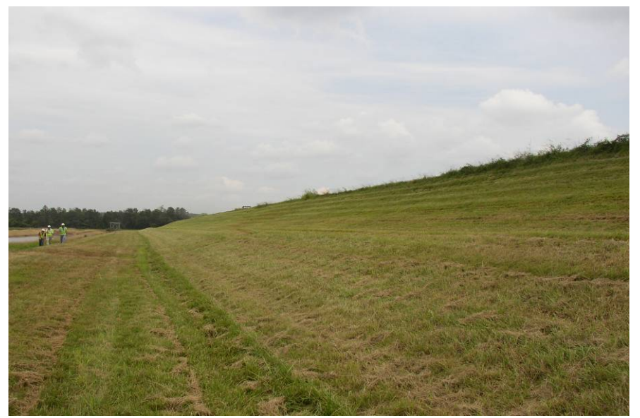
#47 Lower Berm of North Dike – 25-Foot-Wide Berm @ Elev. 625
