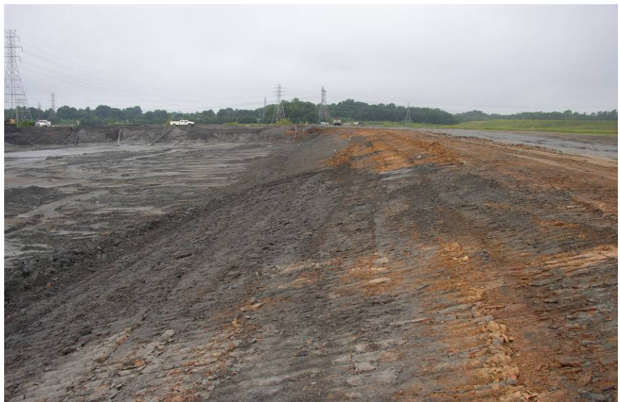
#58 Upstream Slope of Cell 3. Ash Excavated to Depth of About 20 Feet. No Water Impoundment
