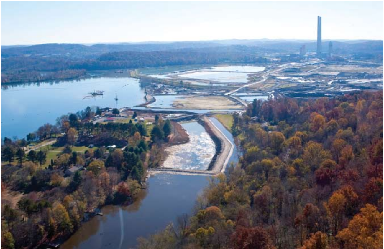
The recovery work on the east embayment has been substantial.
