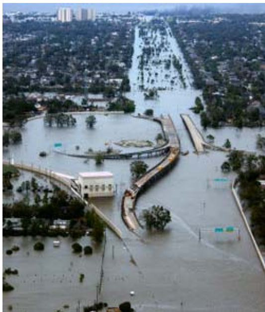
Figure 10 - Flooded I-10/I-610/West End Blvd. Interchange and Surrounding Area of Northwest New Orleans and Metairie, Louisiana
