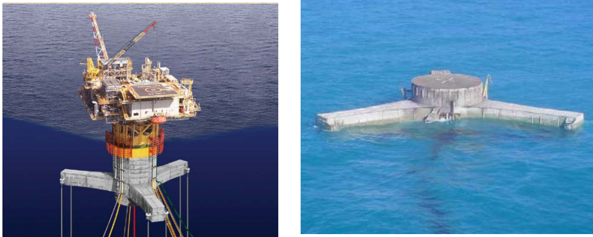
Figure 18 - Typhoon TLP - Pre and Post Hurricane Rita
