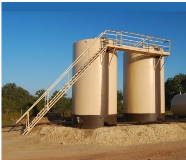
Twin 210 barrel oil tanks inside containment dike
