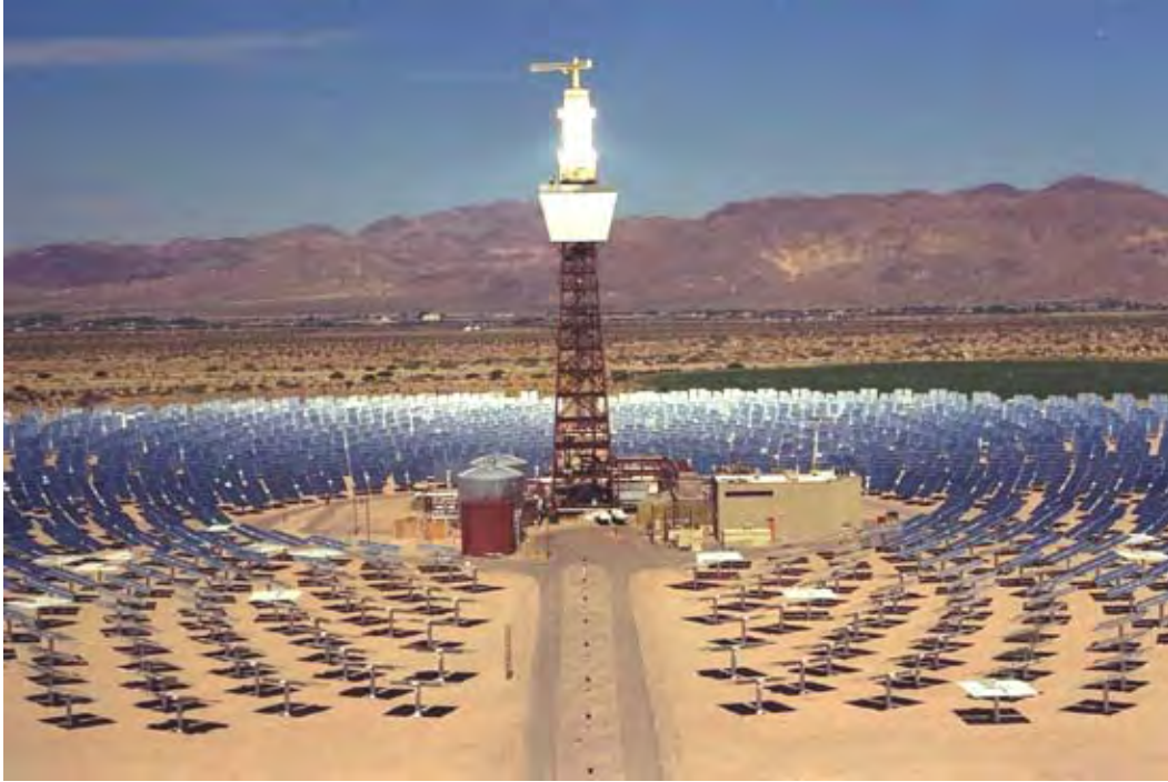
The central receiver of the Solar Two SEGS plant in Daggett, California, glows with sunlight reflected by its circular array of heliostats. (Credit: Joe Florez, Sandia National Laboratories)
