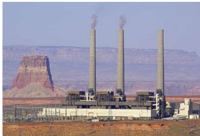
Power Plant near Page, AZ. Photo: iStock.
