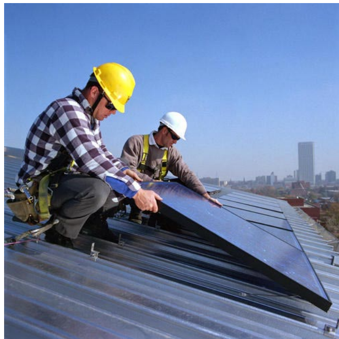
Green workers install solar panels. (Craig Miller Productions and NREL/DOE)
