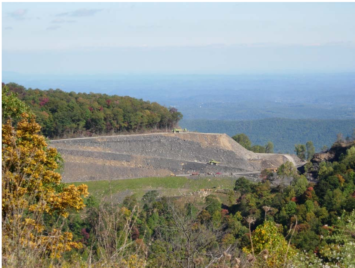
Figure 6.25: Coal Trucks in Tennessee (2006)
