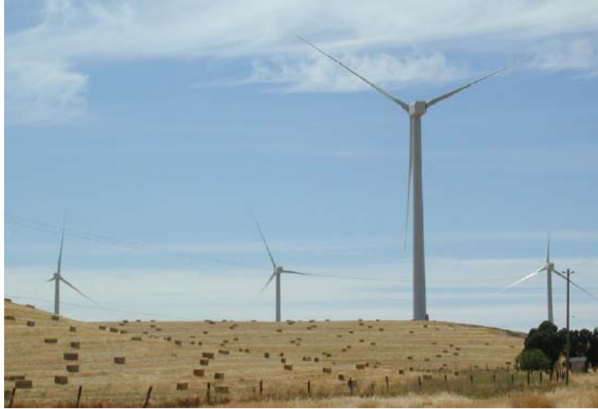
Figure 6.28: Turbines at High Winds Project in Salano, California
