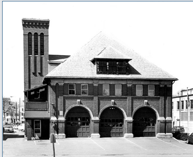
Fire Station, Melrose Town Center Historic District, both a Local and National Register Historic District.
