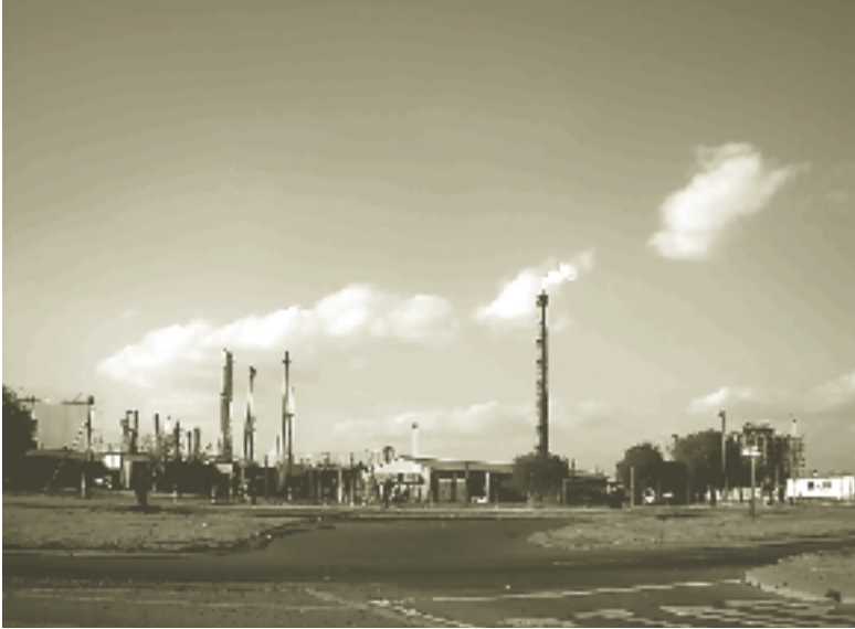
Sasol gas flaring. Such flaring is alleged by environmentalists to be in breach of South African law.
