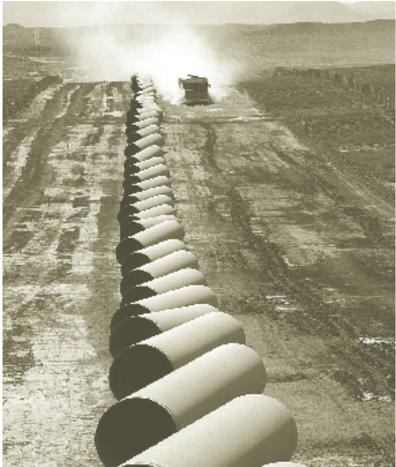
Segments of the Baku-Ceyhan pipeline await assembly.
