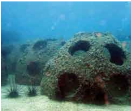
Reefballs placed to establish an artificial coral reef at Royal Pahang Reef, Pulau Renggis, Tioman, Malaysia. Photo: Debby Ng
