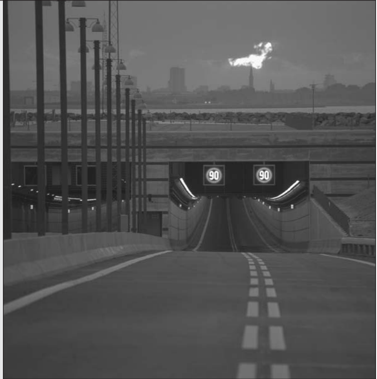
Oresund Bridge tunnel connecting Sweden and Denmark (both photos courtesy of Oresund Bridge Project)
