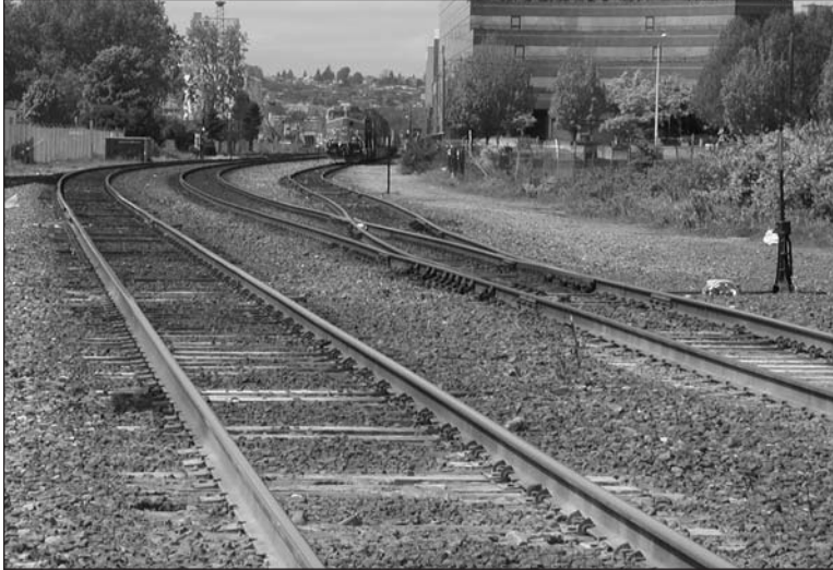
Burlington Northern/Santa Fe railroad tracks along the central waterfront
