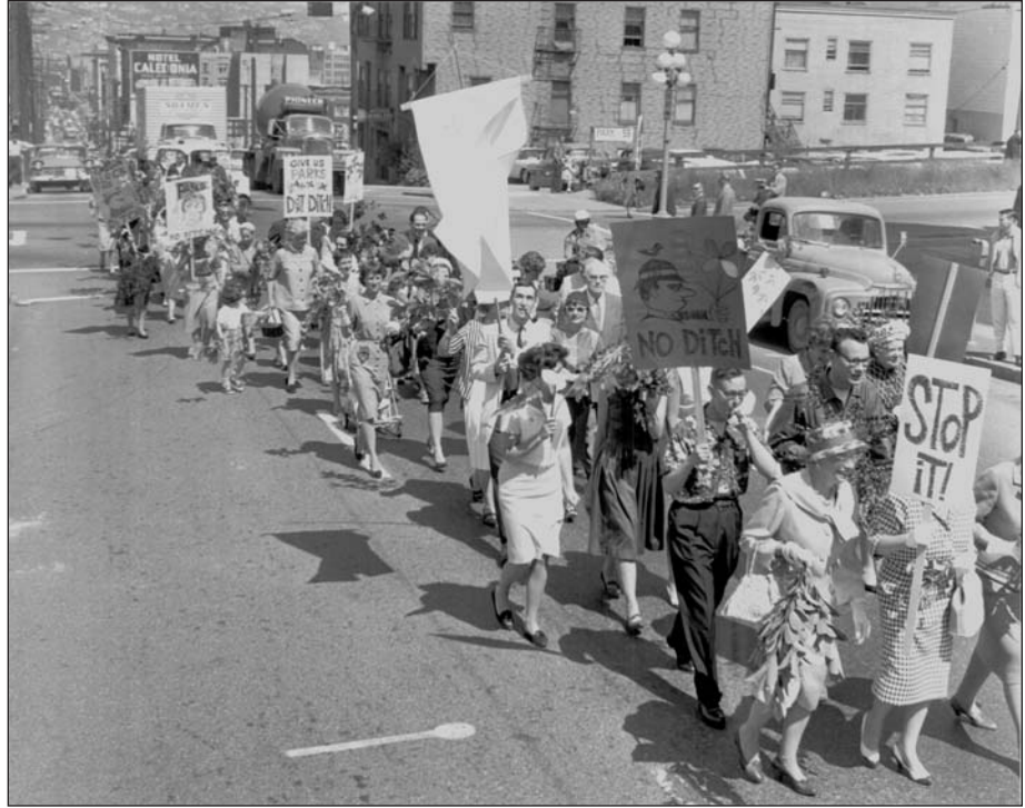
Before construction of I-5: Citizens march along the prospective I-5 route in downtown Seattle, protesting against an unlidded freeway trench (courtesy of MOHAI)
